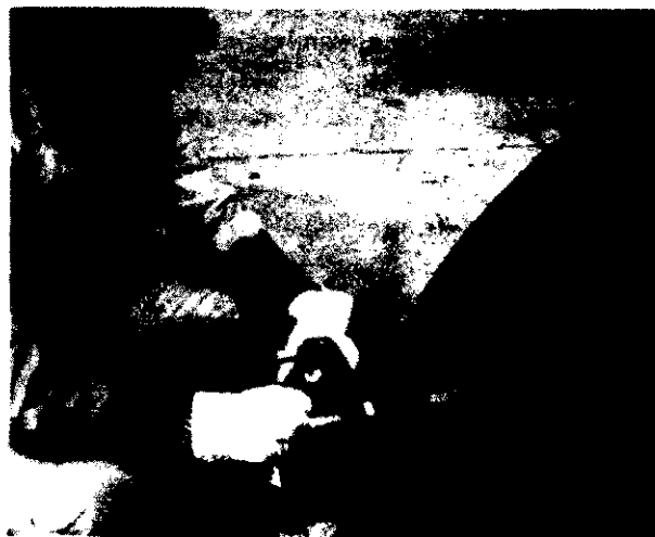
Fig. 14-7. Aligning a flange using a level, when the pipe is known to be in a horizontal position.
